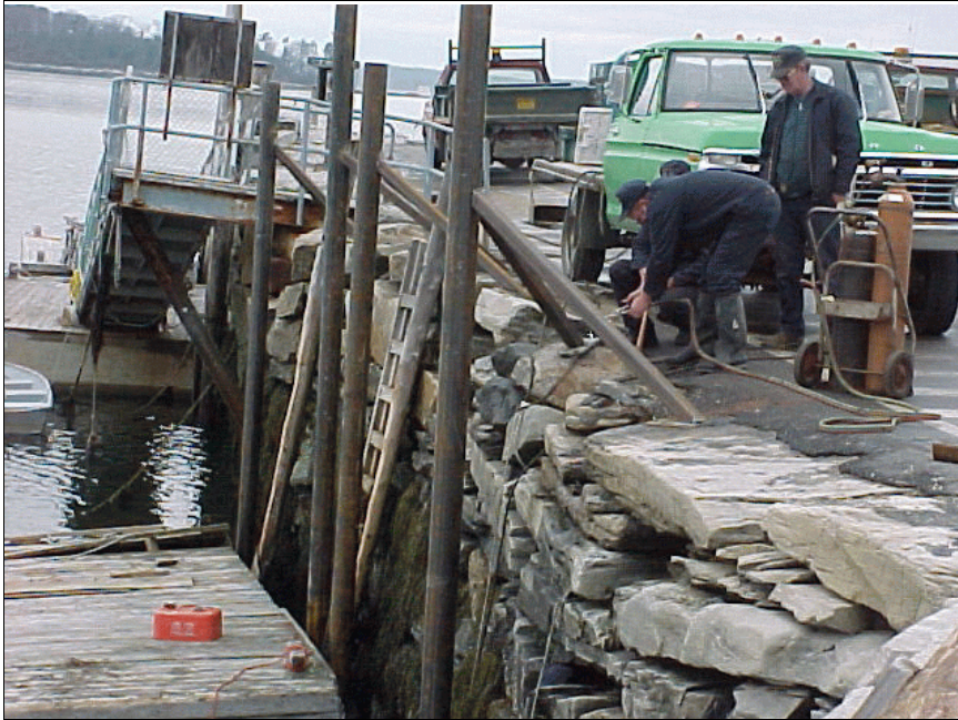
Installing new punt floats at the Stone Wharf
