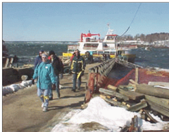
Chandler's Cove Wharf under reconstruction on a very stormy day
