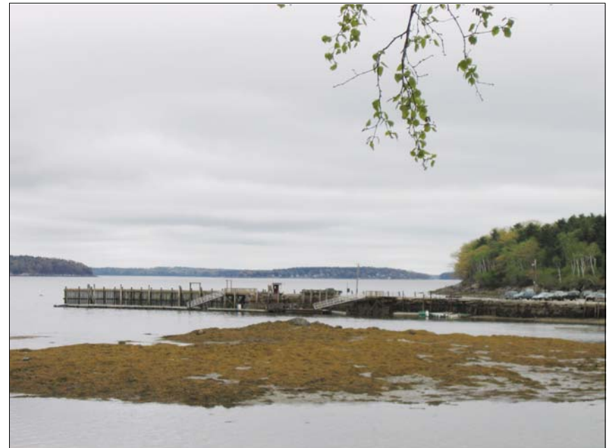
The expanded Stone Wharf at low tide
